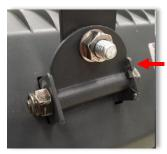
Heater bracket installed outside upper tab.
